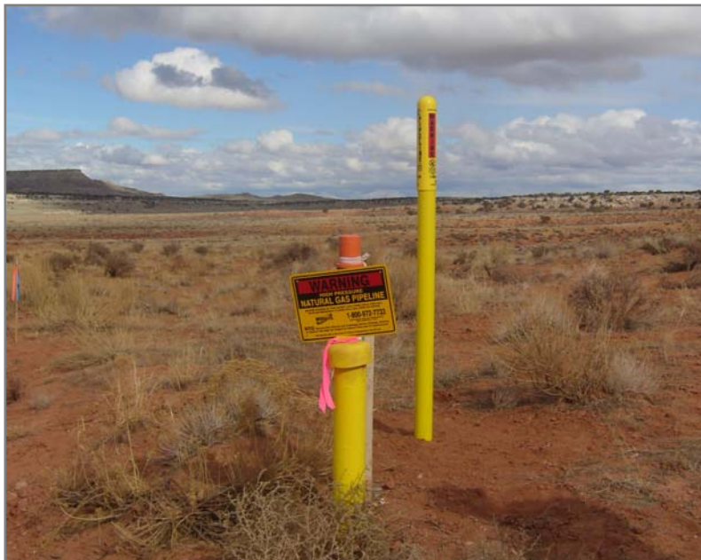
Figure 5: Williams gas Transmission Pipe location
